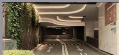
Basement slope climbing
